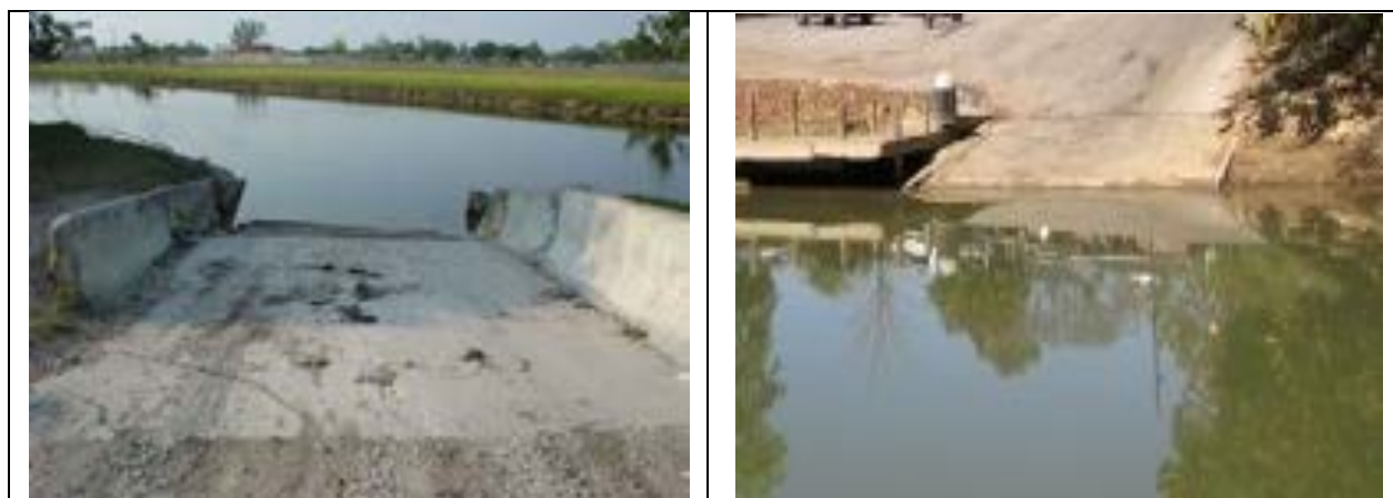
Figure 5: Typical view of ramps
