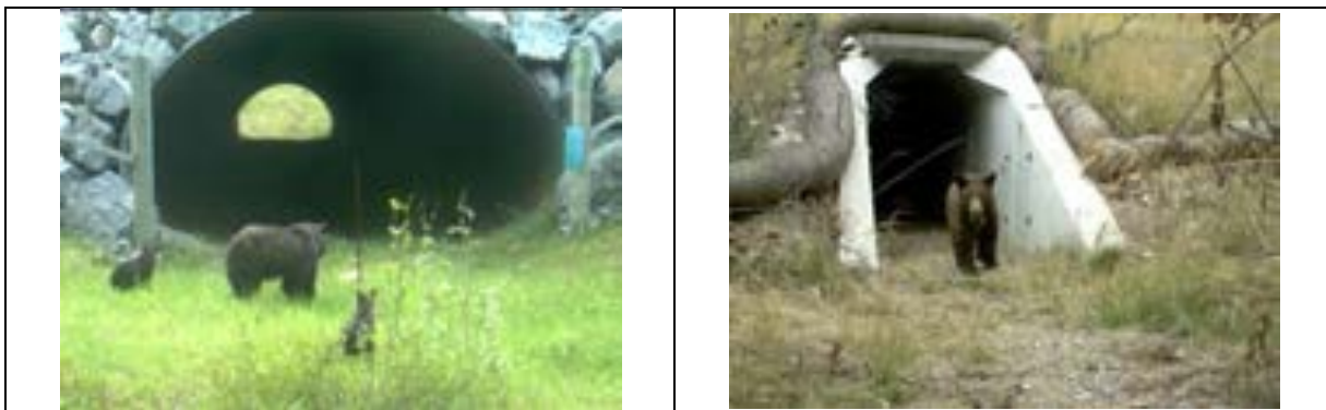
Figure 2: Typical view of culvert
