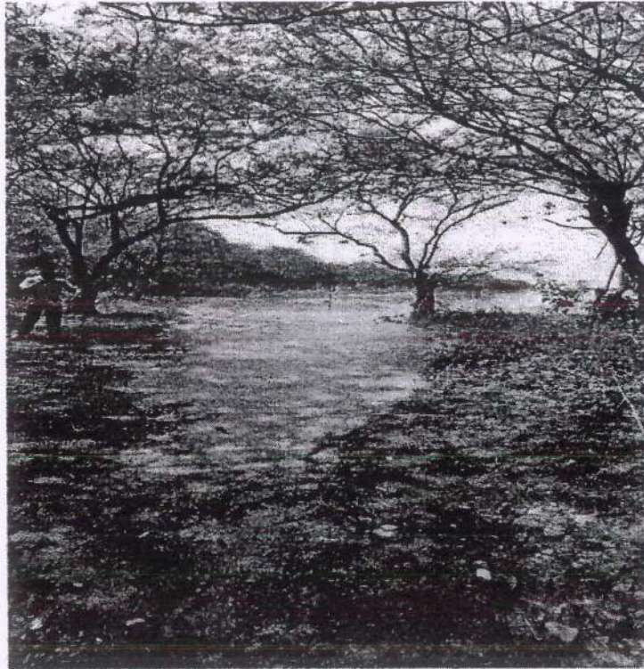
Water is at present over flowing from the propose fuse plug area. The dam is at full capacity
