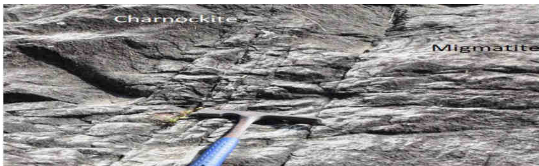
Fig. 17. Valanthode SHEP: Two sets of Joint planes in dam axis
