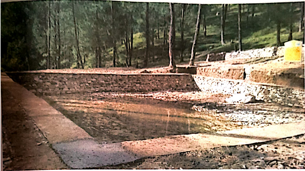
Water Harvesting Tank
