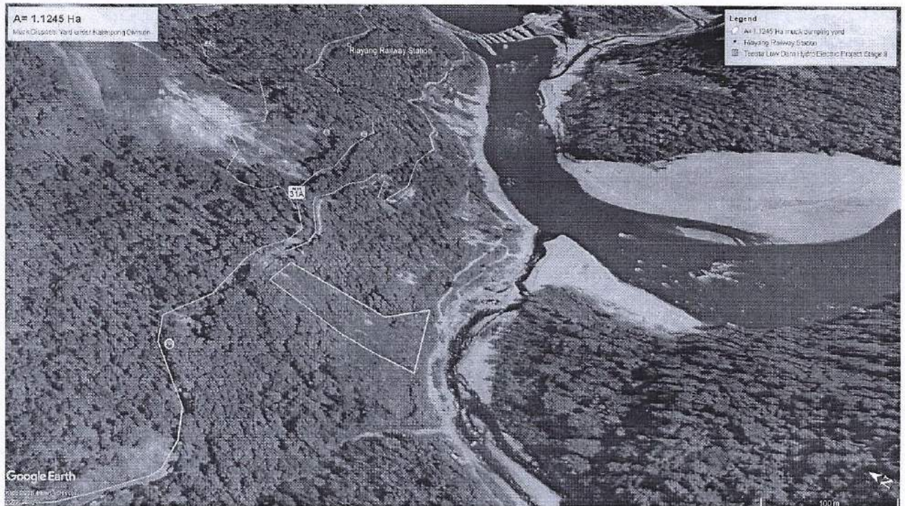
Figure- 6: Muck Disposal Yard KML
