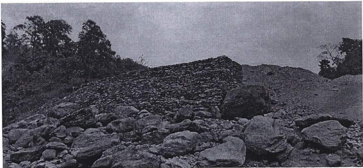
Figure- 1: Erected Gabion wall surrounding the periphery of muck disposal site
