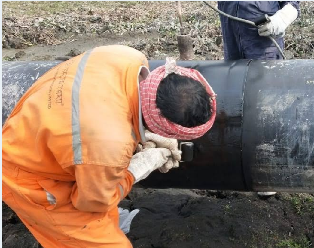
Figure: Joint coating for insulation in the exposed pipe joints
