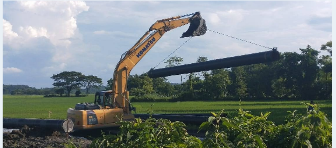
Figure: Stringing of pipes along RoU
