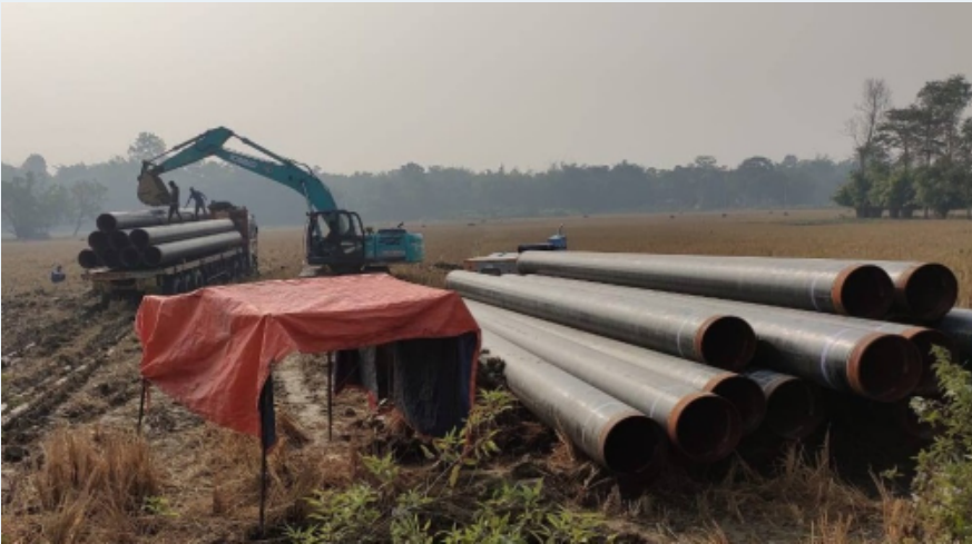
Figure: Unloading and stacking of pipes
