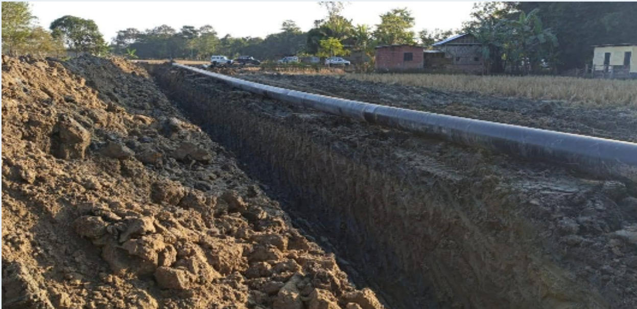
Figure: Trench excavated along the pipe string on RoU
