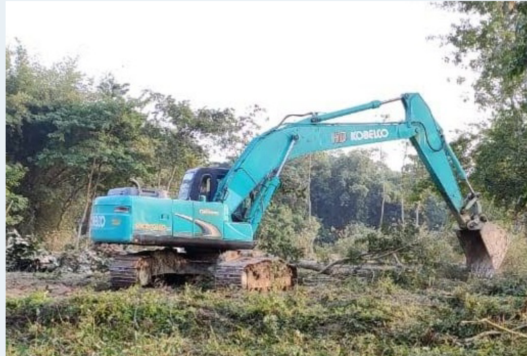
Figure: Both the images showing grading of top soil along the RoU
