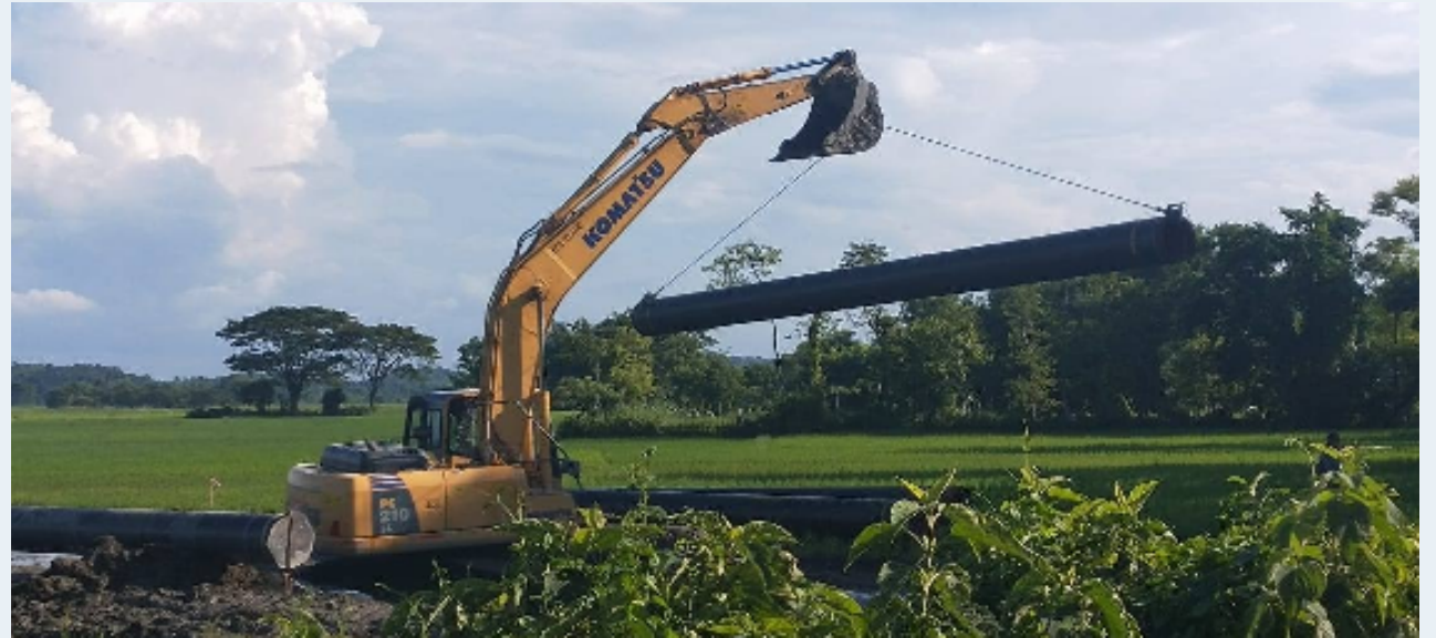
Figure: Stringing of pipes along RoU
