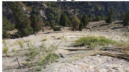
Reclamation Works completed at DS-8
