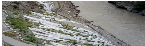
Reclamation Works completed at Power House Site DS-3
