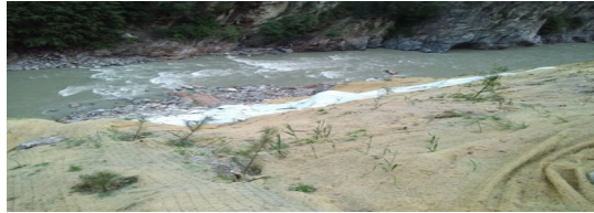
Reclamation Works completed
