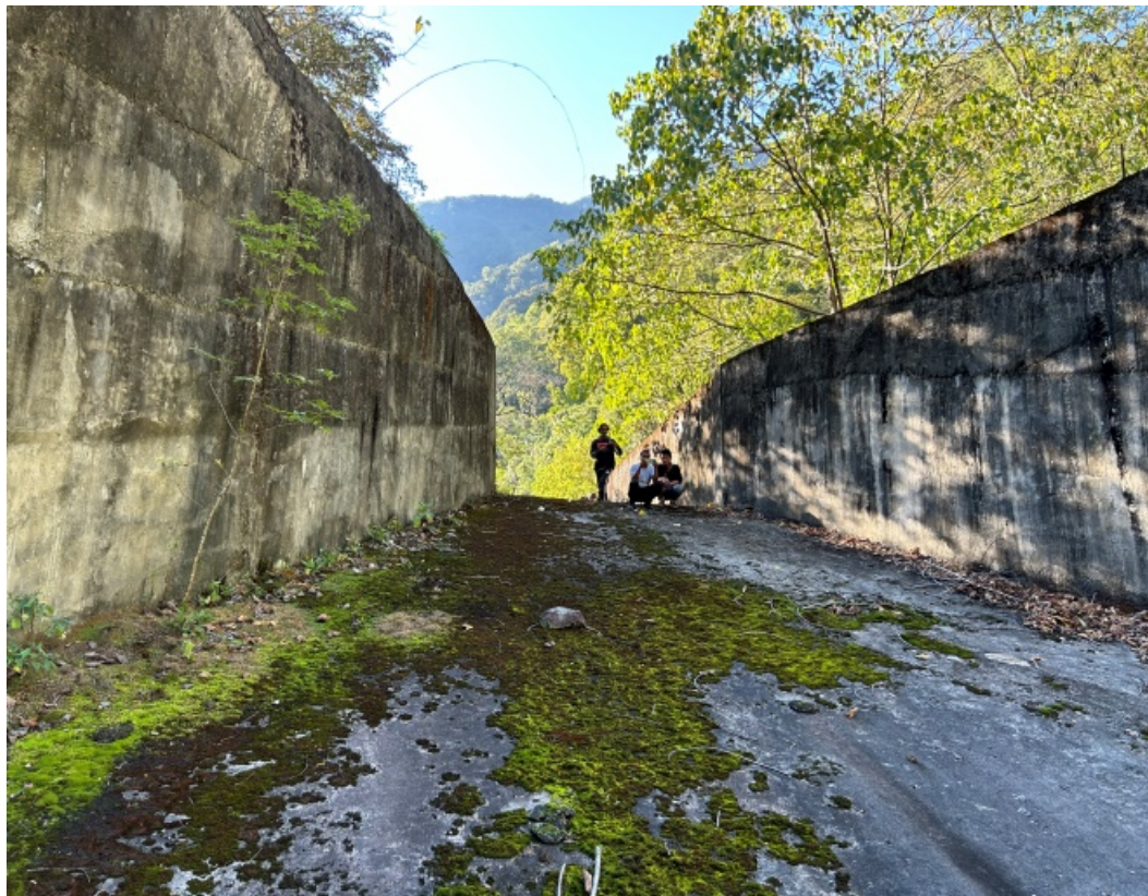
Fig. 17 A view showing the existing D- Tank
