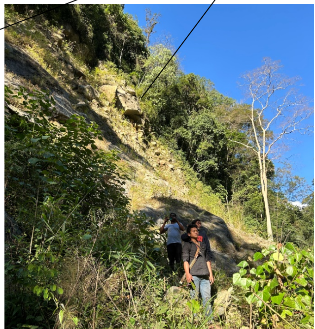
Fig. 14 Views showing the slide at right abutment of Barrage Axis
