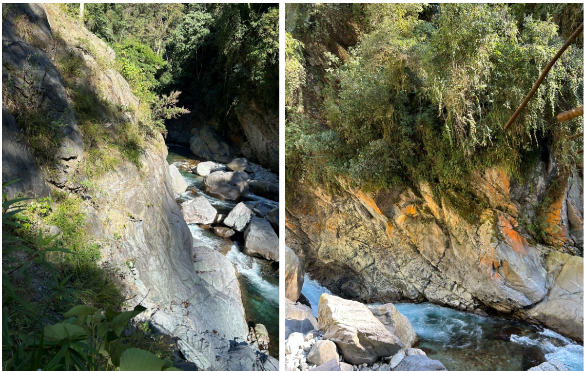
Fig. 11 A View showing rock exposure on the (a) Right Bank (b) Left Bank
