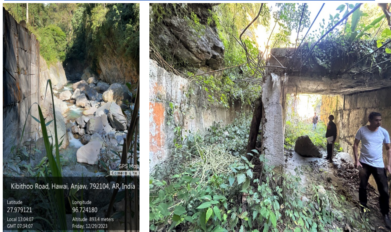
Fig. 15 View showing the existing Intake structure
