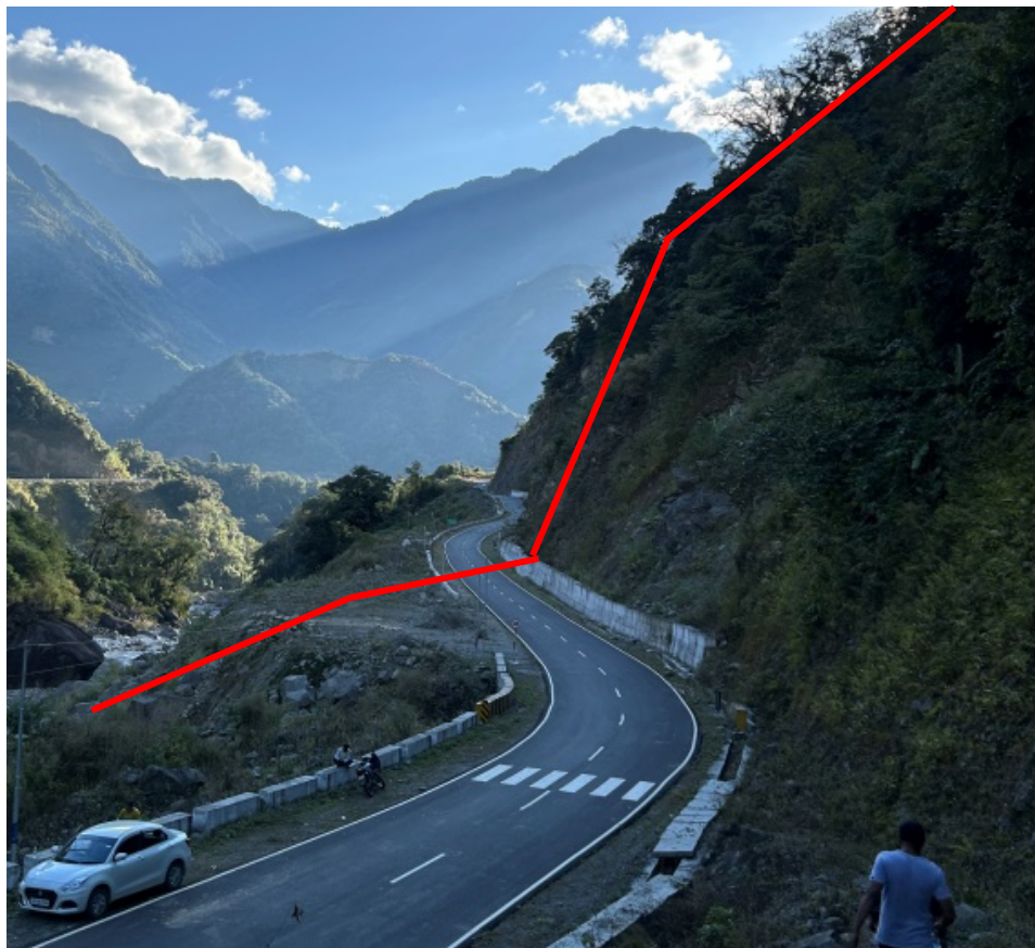
Fig. 20 A view showing the hill slope for Penstock Alignment
