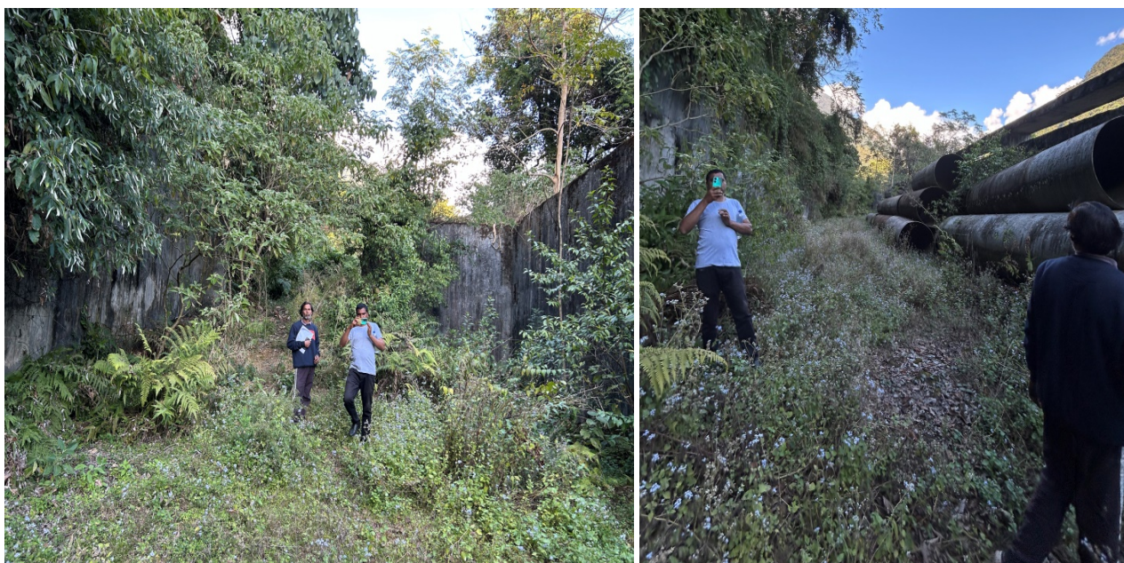
Fig. 19 Views showing the existing Forebay Tank area
