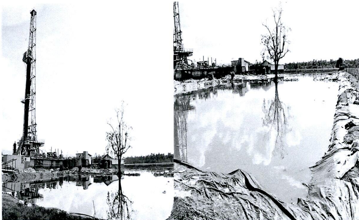
Fig. 2: A typical waste pit secured with HDPE lining
