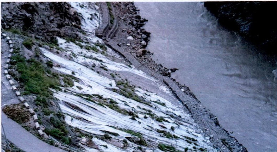
Reclamation Works completed on DS-3
