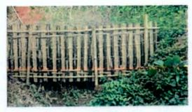
plugging when assembled like a box and situated in the gully. Soil and/or fallen tree leaves are put into the box to arrest the sediment from flow downstream in the gully valley. The local bamboo can be used for lattice bars of the brushwood. The estimated budget for construction of the brushwood check dam is 2.5 lakhs.
