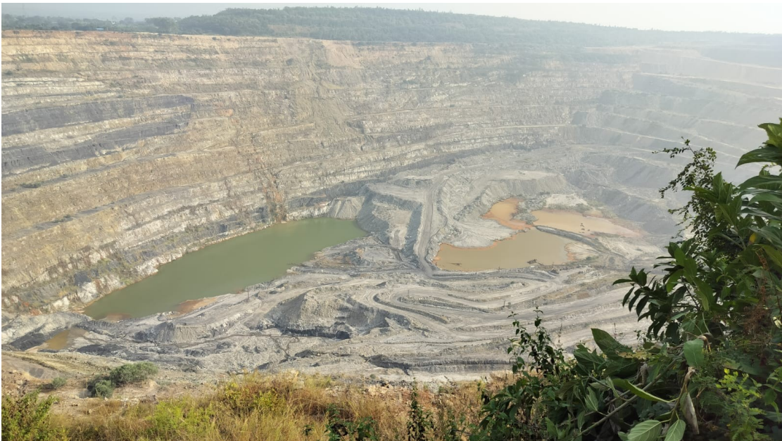
Photos showing GKOC void areas without Safety Zone.
