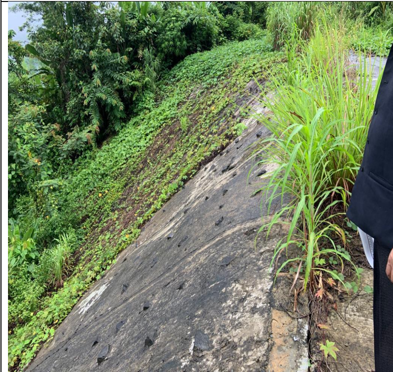
Culvert allowing Stream to flow
