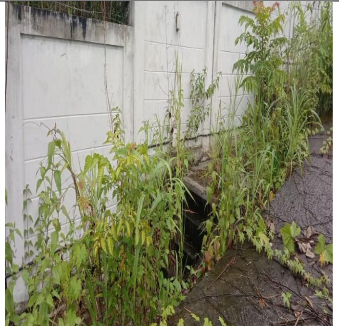
RCC Boundary Wall
