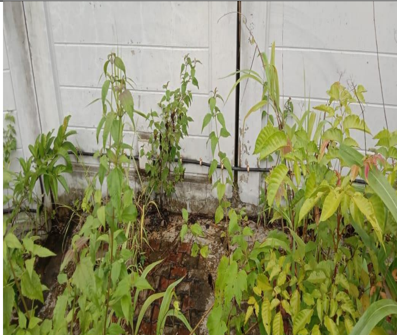
RCC Boundary Wall
