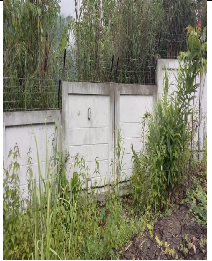
RCC Boundary Wall
