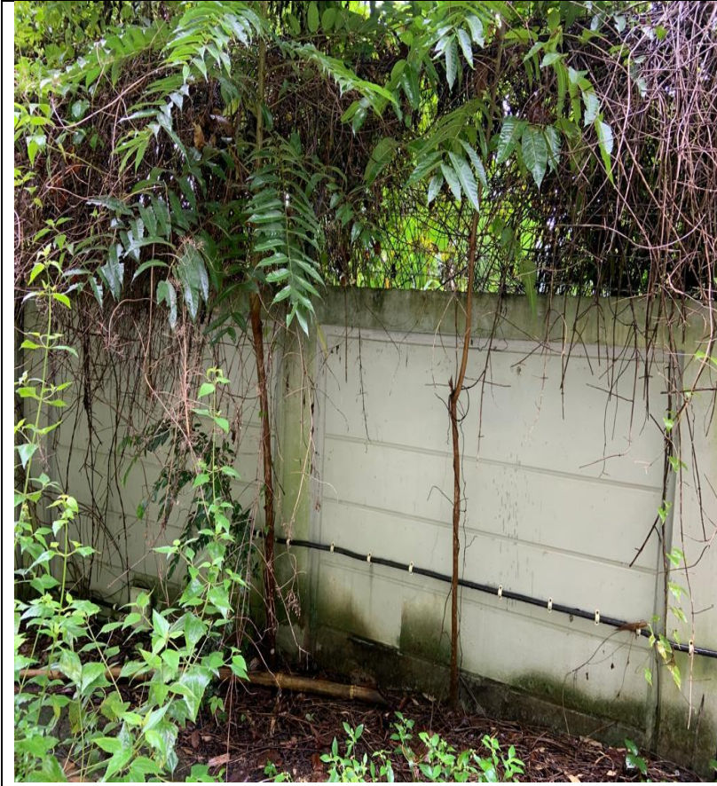
RCC Boundary Wall
