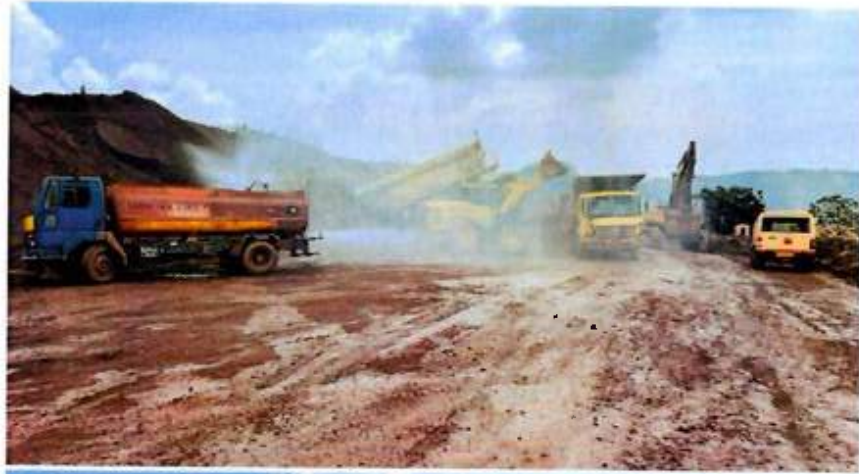
Plate-25 Sprinkling water on mining road to suppress dust
