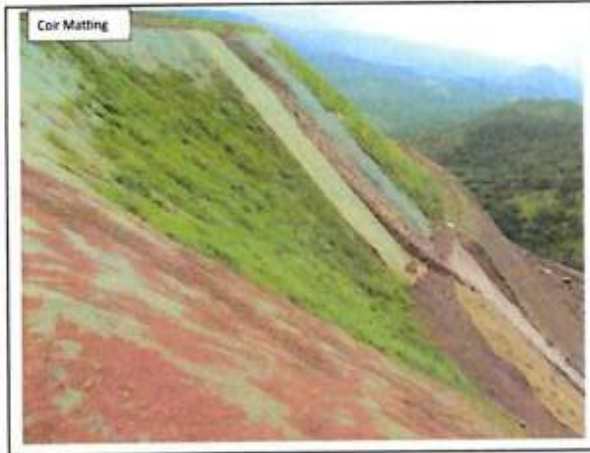
Stabilisation of the waste dump slopes
