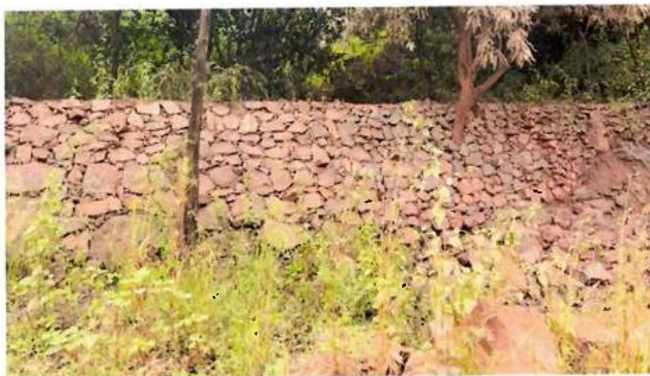
Retention wall to prevent soil erosion
