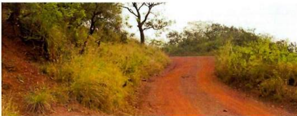
KSMCL-TIOM road inside the lease area
