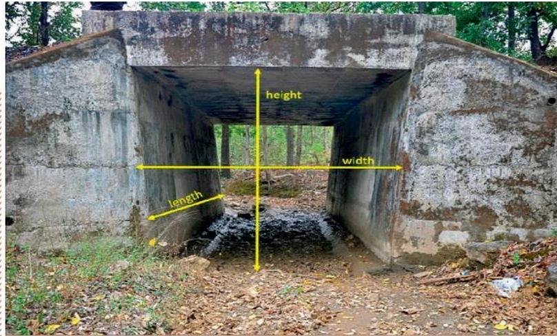
Figure 7.1. Dimensions of an underpass determining its openness. Source: Photograph by Akanksha Saxena.
