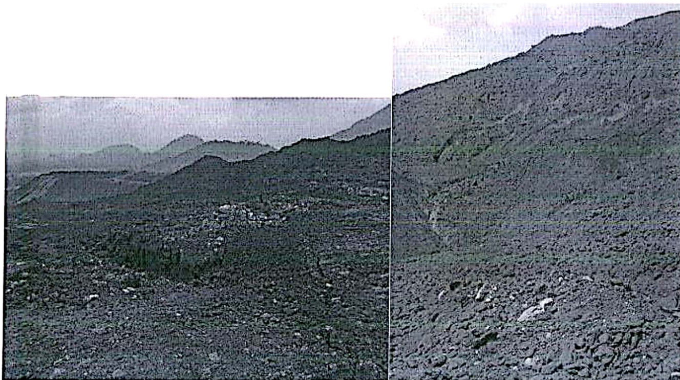
Figure 5: Photograph of red mud disposal by dry stacking methodology
