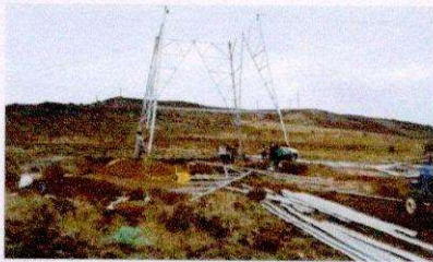
Tower Erection in progress
