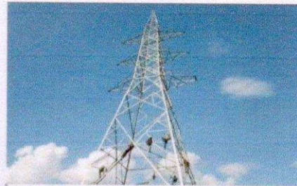
Cross Arms Erected
