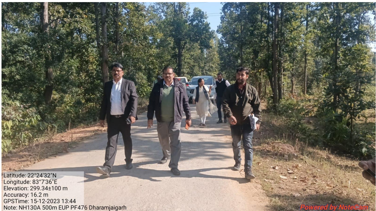
Site- 6 PF-476, 2 Elephant Underpasses (EUP) lenth (240+150M), at Village Khadgaon and Koilar, lanth of proposed road in this section is 2.6 Km towards Pathalgaon.
