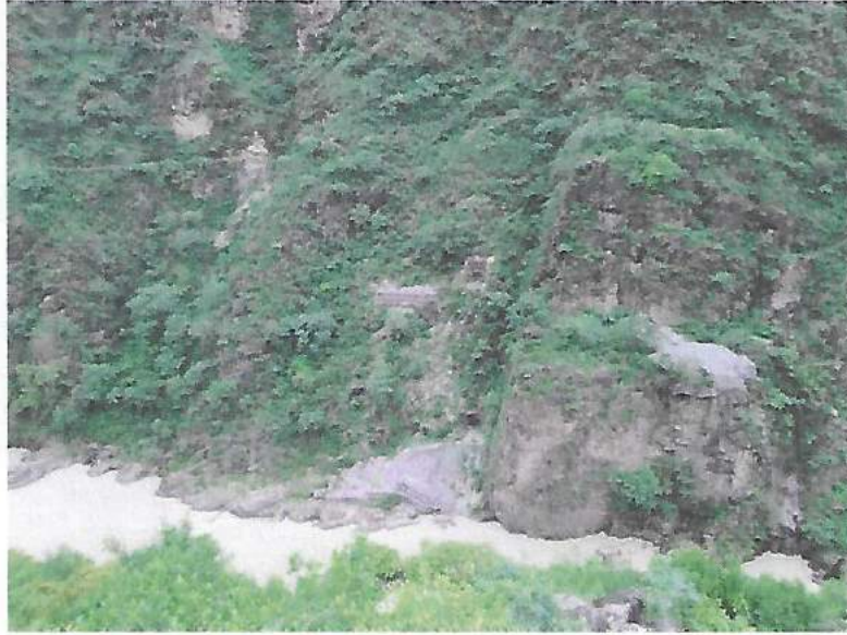
Power House Intake Site
