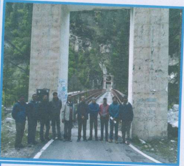
Sukhrali Bridge (To be Submerged)
