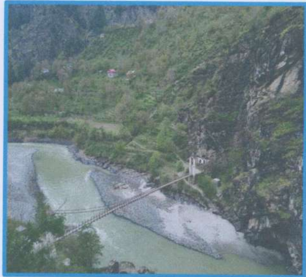
Borrow Area (River Bank Mining)
