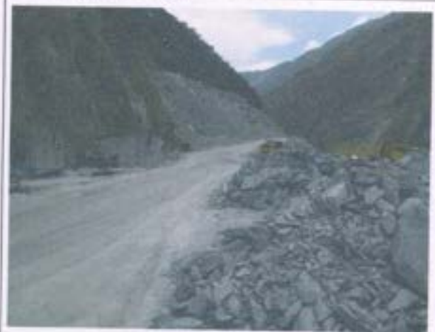
Road to Barrage
