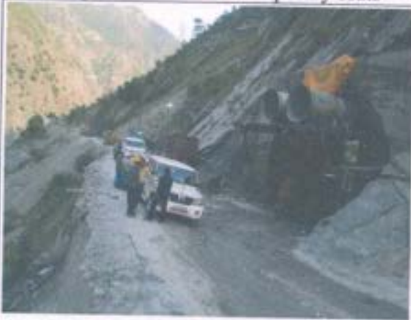
Tunnel for Power Hose
