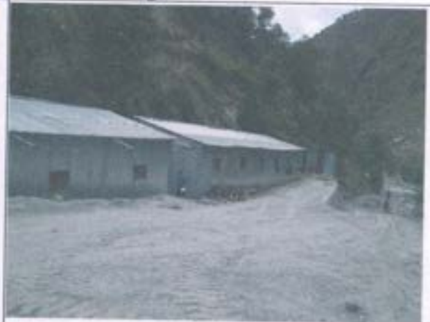
Temporary Labour Hut
