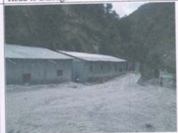
Temporary Labour Hut
