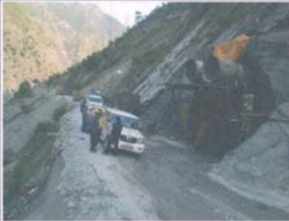
Tunnel for Power Hose
