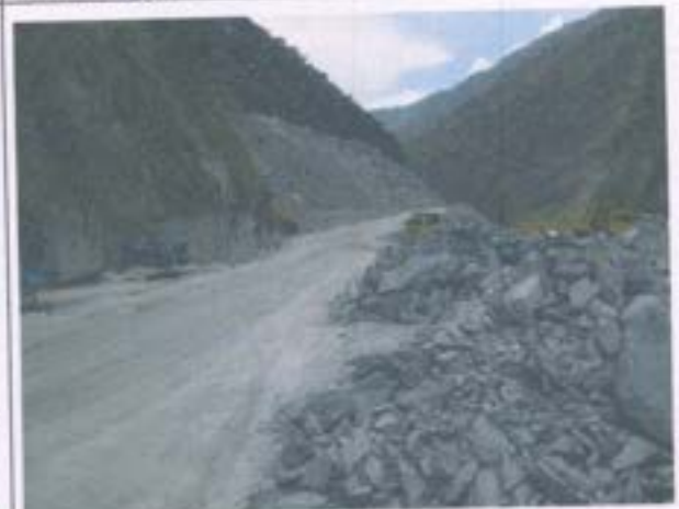
Road to Barrage
