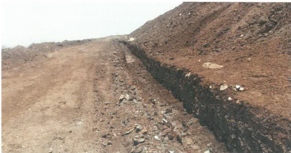
EARTHEN GARLAND DRAIN AT DUMP
