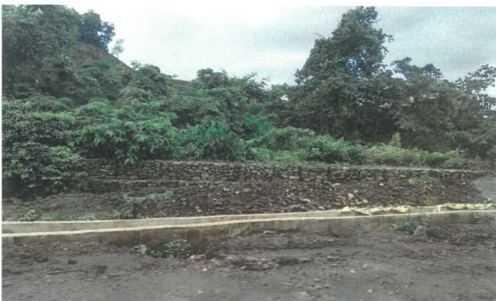
CONCRETE DRAIN AND CREATOR BOULDER WALL AT BASE OF OB DUMP
