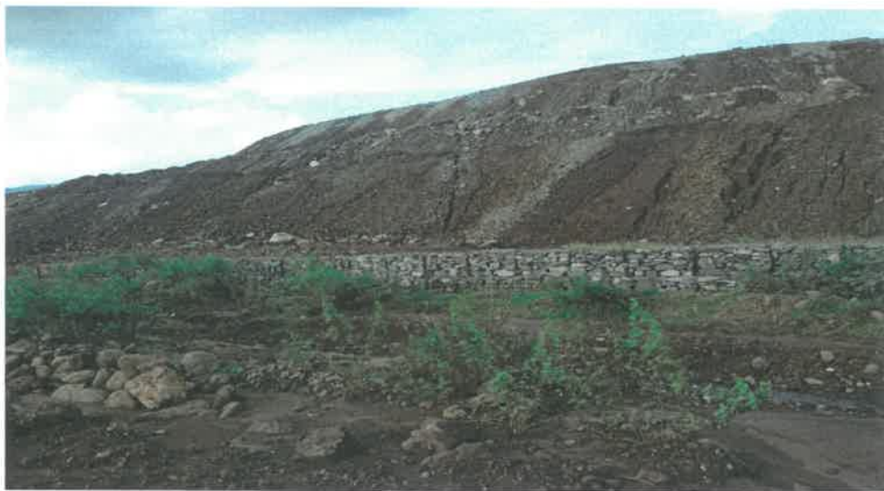
GARLAND DRAIN AND CREATOR BOULDER WALL AT BASE OF OB DUMP
