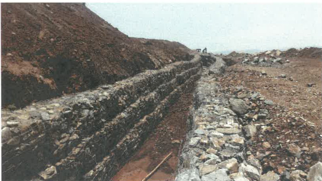
CREATOR BOULDER WALL DRAIN AT OB DUMP
