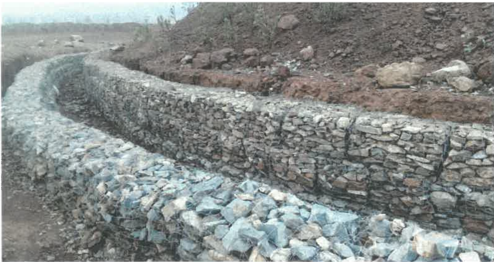
CREATOR BOULDER WALL DRAIN AT OB DUMP
