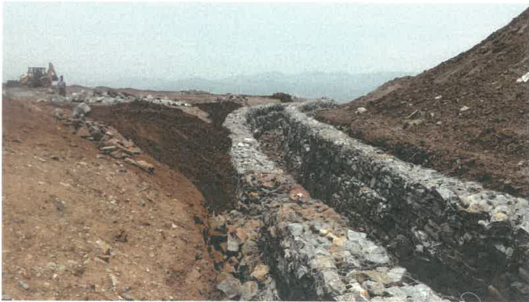
CREATOR BOULDER WALL DRAIN AT OB DUMP
