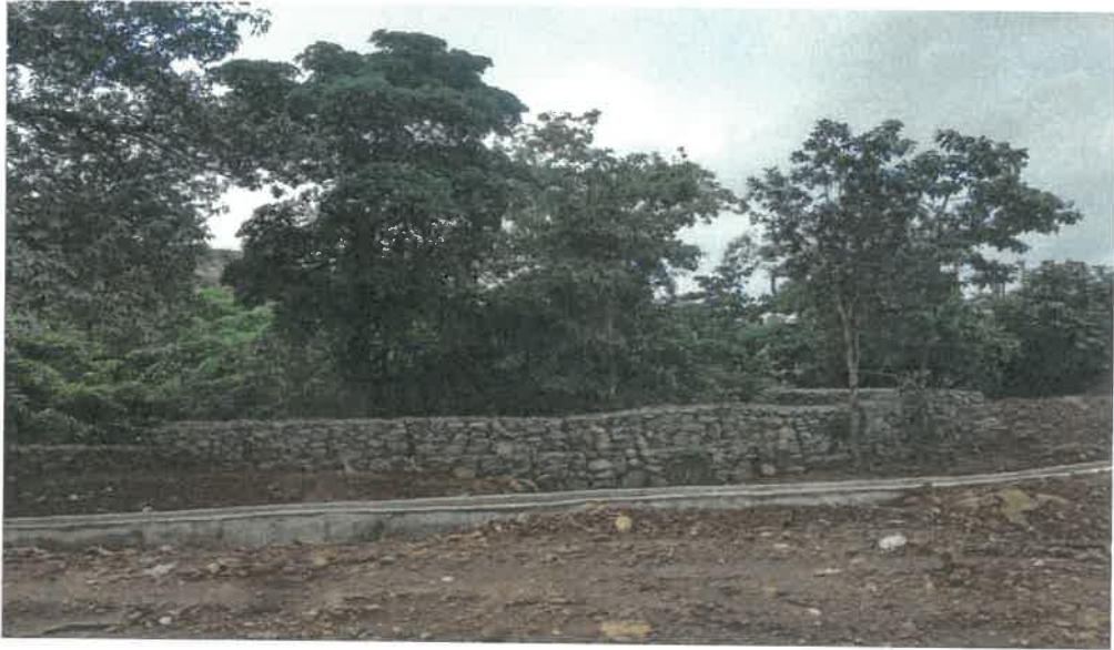
CONCRETE DRAIN AND CREATOR BOULDER WALL AT BASE OF OB DUMP
