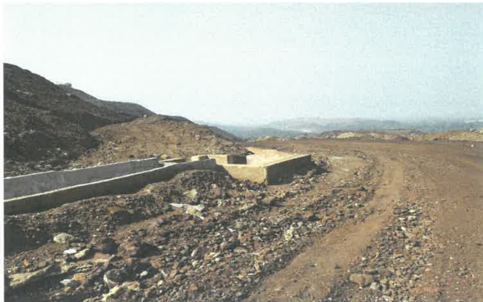
ROAD CROSSING WITH HUME PIPE AND COLLECTION CHAMBER
