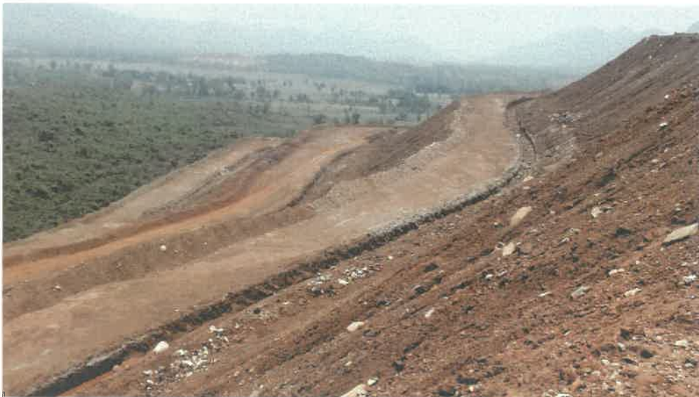
EARTHEN GARLAND DRAIN AT DUMP
