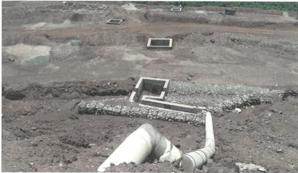
PIPE LINE ARRANGEMENT WITH VAT AT THE SLOPE OF THE DUMP
