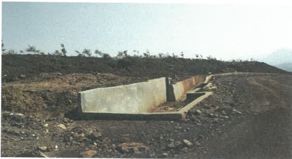
ROAD CROSSING WITH HUME PIPE AND COLLECTION CHAMBER
