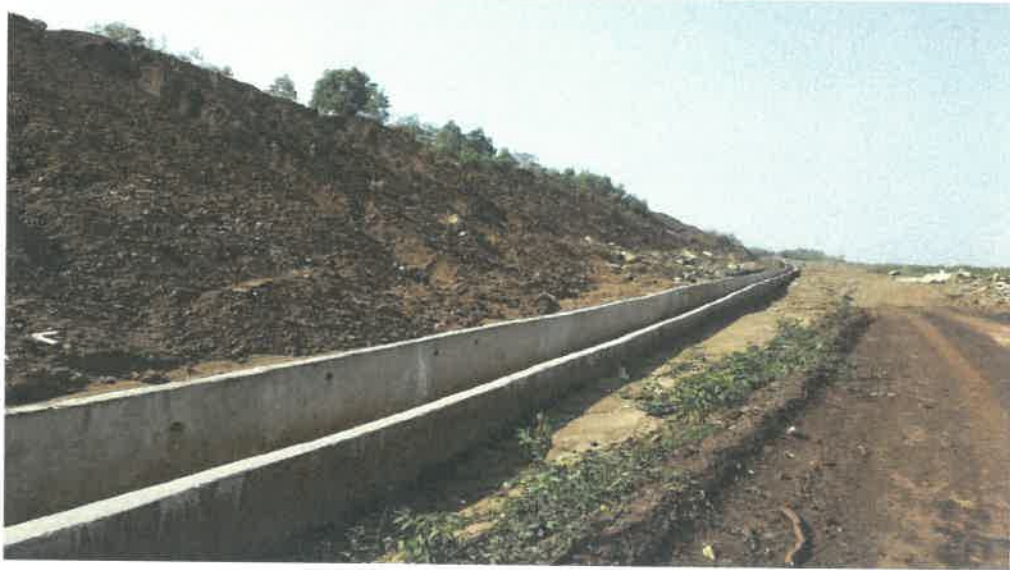
CONCRETE DRAIN FROM TOP TO BOTTOM OF THE OB DUMP
