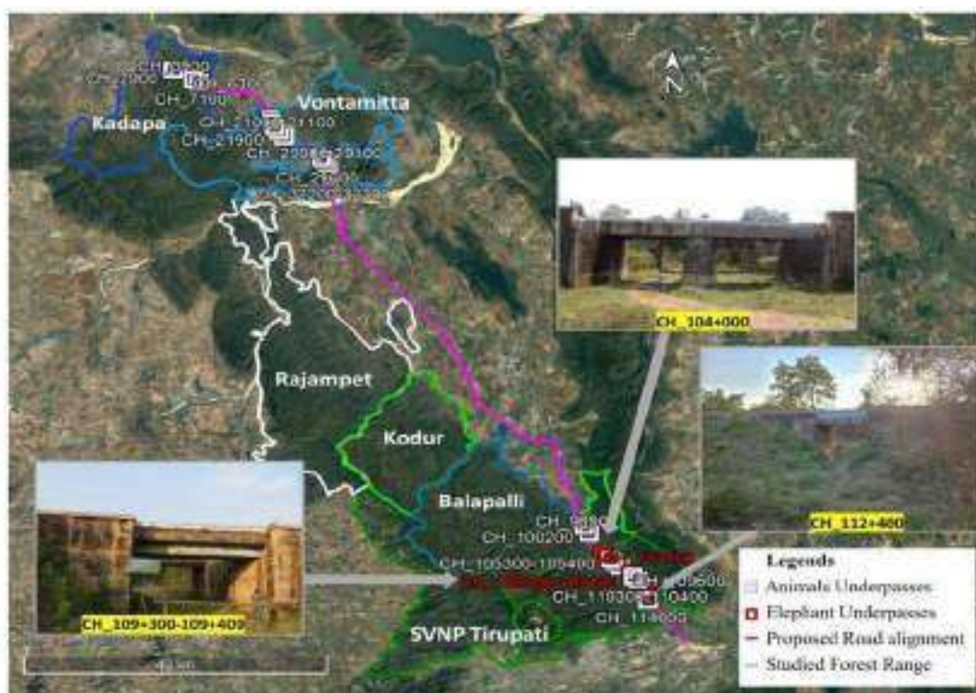
Figure 15: Photographs showing the identified railway underpasses for elephant corridor along adjacent proposed elephant underpass of the proposed alignment.
