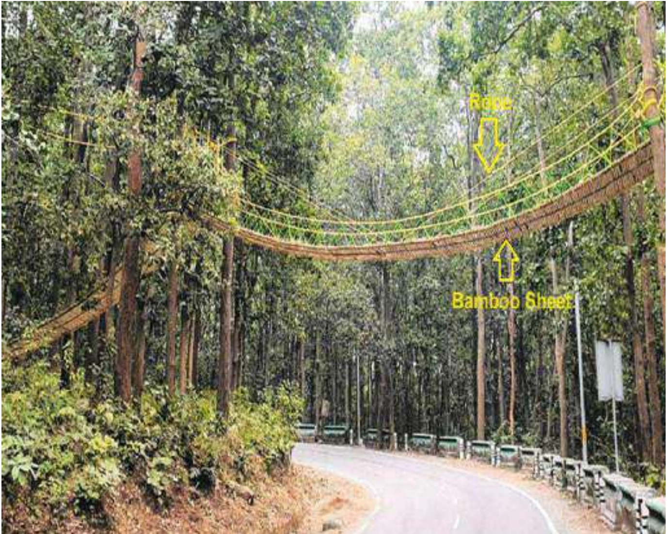
Figure No (a): An illustration of the artificial bridge suggested on the project road
