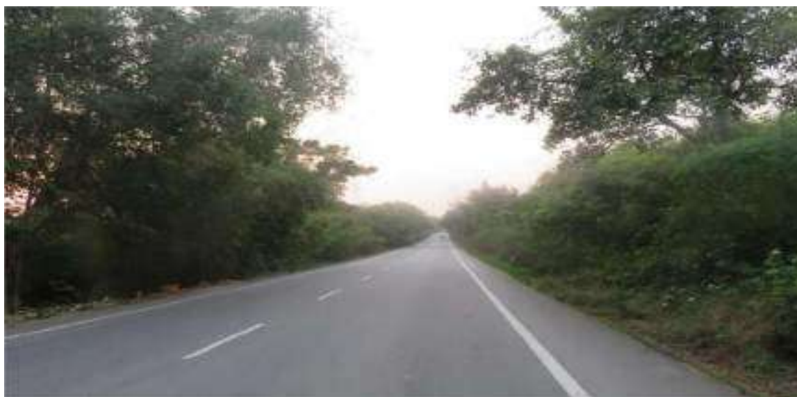
Figure 8: A view of existing highway to the proposed alignment.
