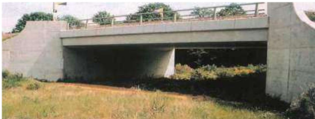
Figure 16: Example of an underpass below highway (Photo source: Google images).
