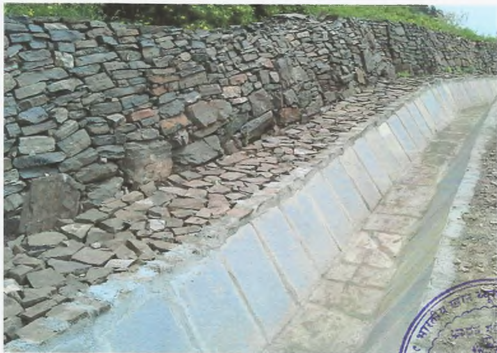
LOOSE BOULDER TOE WALL AND GARLAND DRAIN
