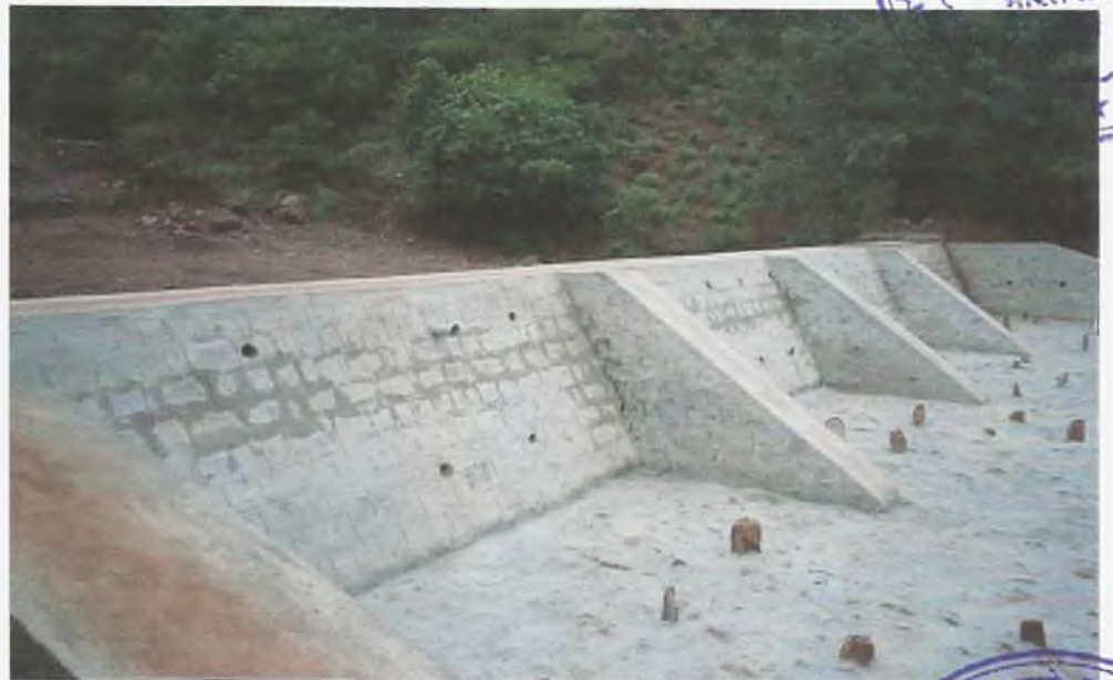
STONE MASONRY CHECK DAM - SMCD
