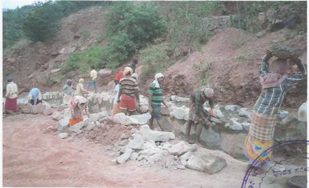
LOOSE BOULDER CHECK DAM & TOE WALL TW-1 In progress
