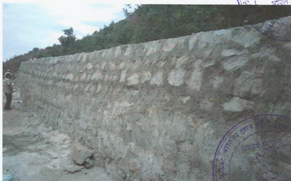
TOE WALL TW-1 (In progress)
