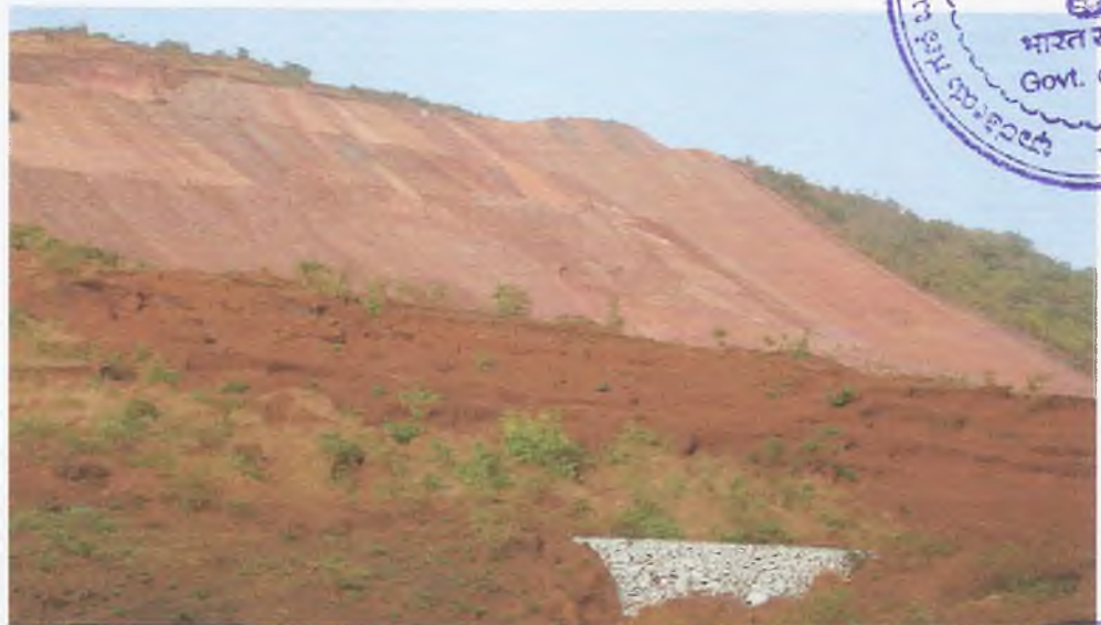
STEP DUMPING AND GULLY CHECK
