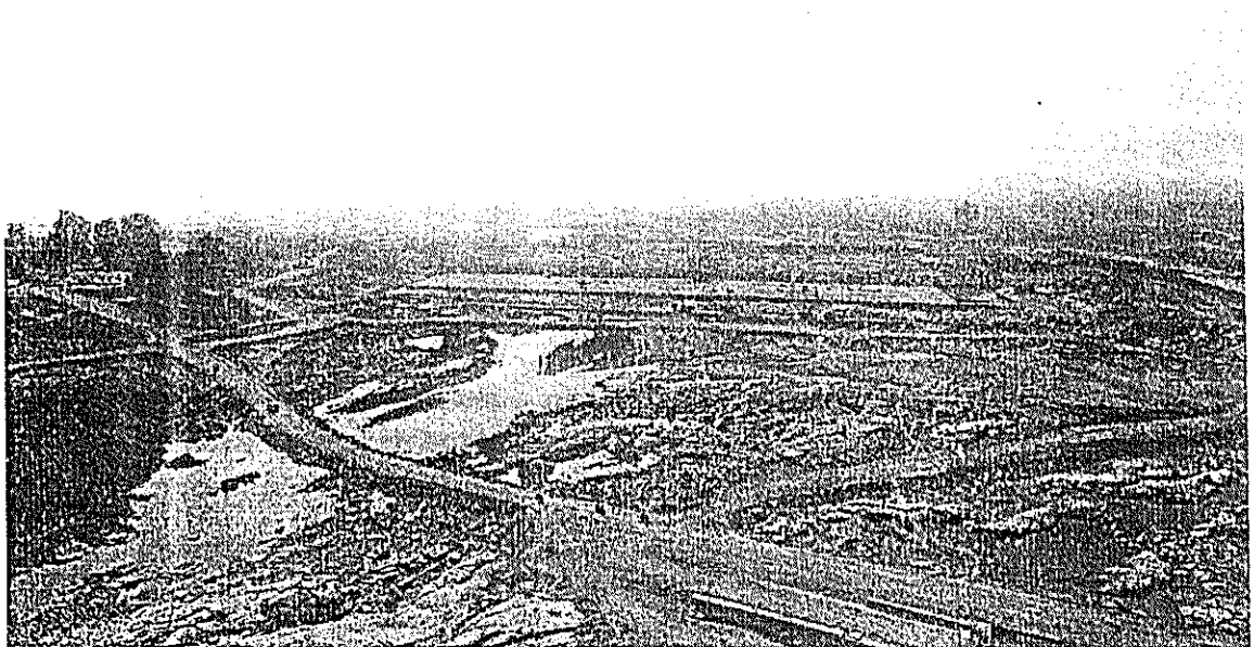
PHOTOGRAPHS OF PROJECT SITE
