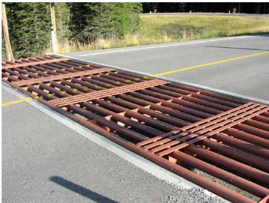
Fig. 4: Cattle guards/grids to be installed at both ends of the underpasses and fenced sections
