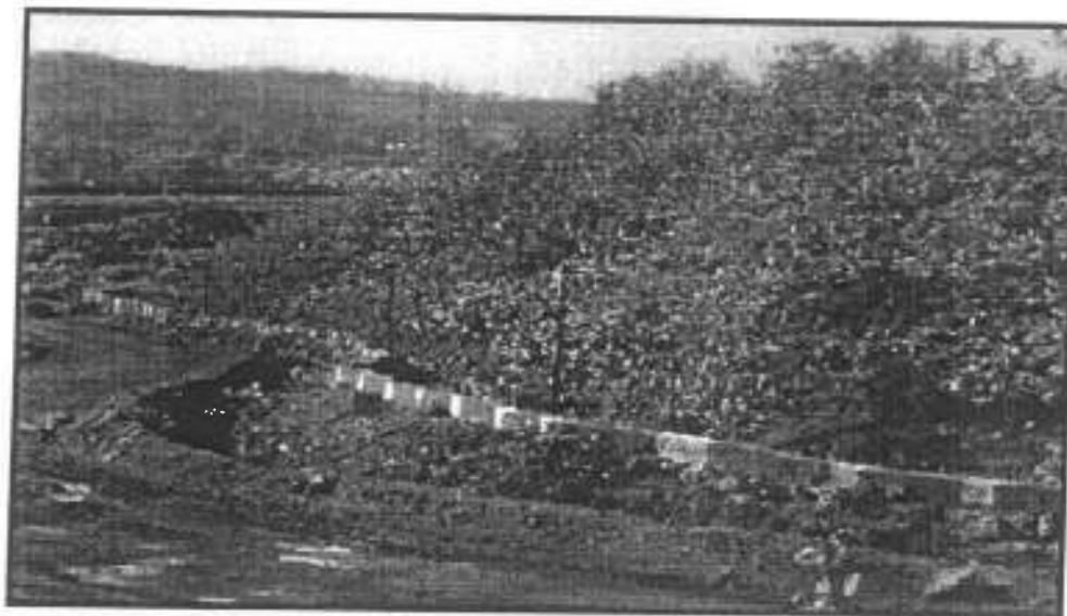
Garland Drain around Waste Dump
