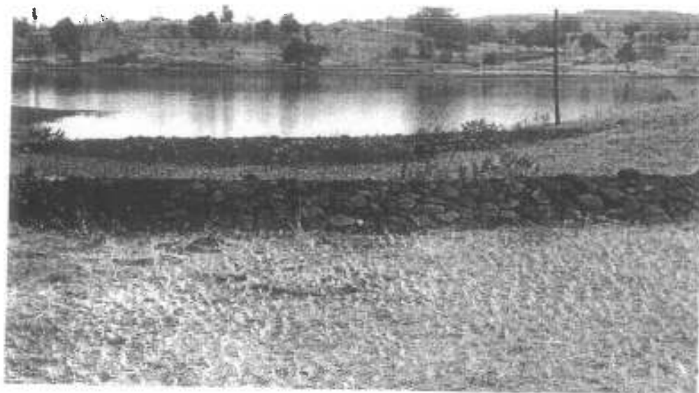
Loose Boulder Structures
