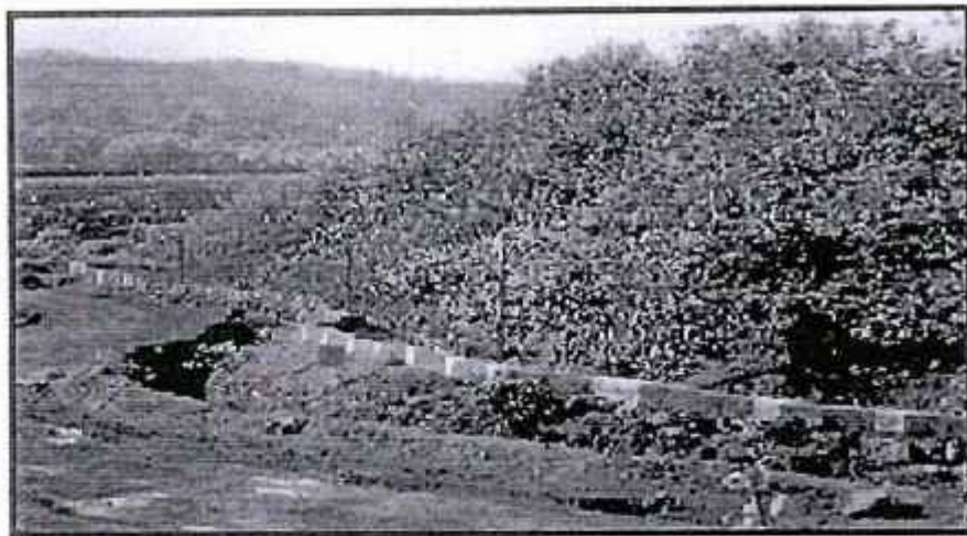
Garland Drain around Waste Dump
