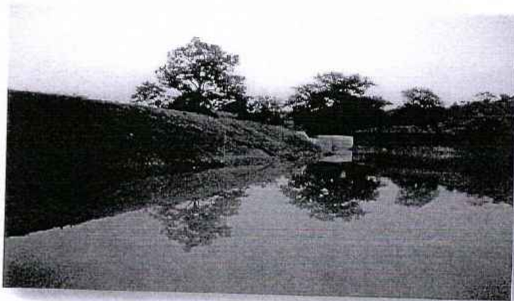
Check Dam to restrict Soil erosion & silt flow
