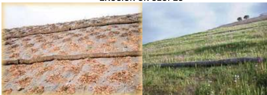
FIG 6: APPLICATION OF COCO FILTERS FOR CONTROLLING SOIL EROSION ON SLOPES
