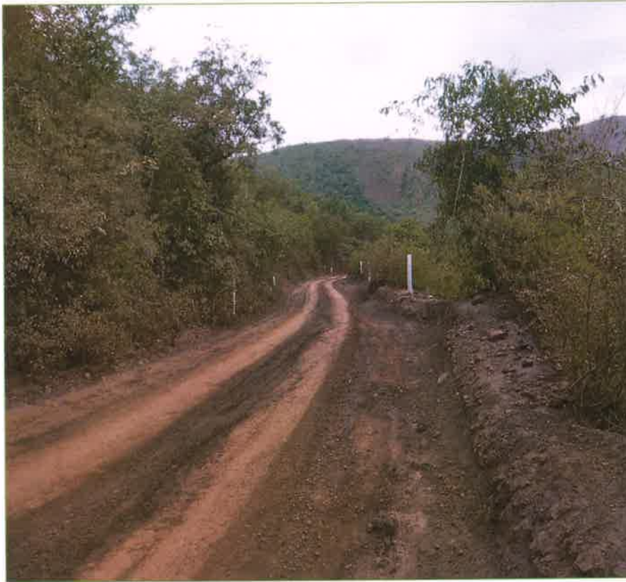
Annexure-IV: Reinforced Cement Concrete Pillars demarcated on the forestland to be diverted
