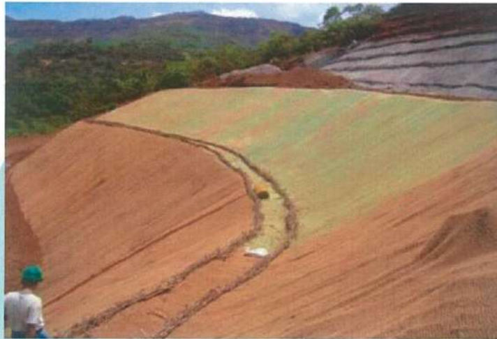
Fig 6.10: Geotextile Application
