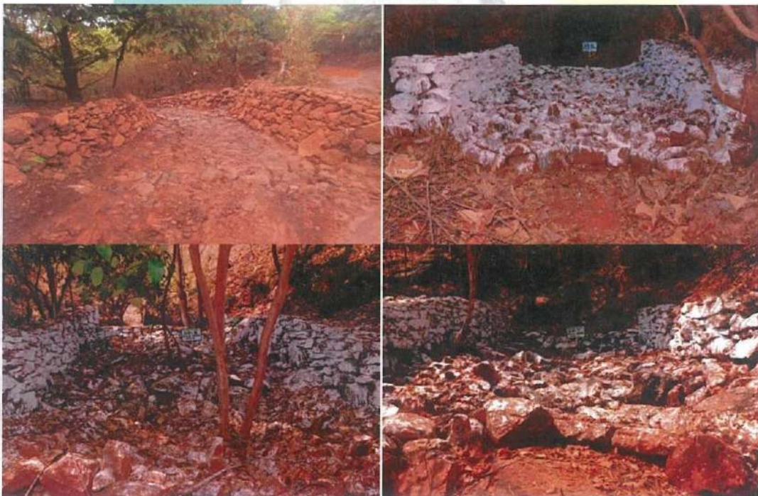
Fig 6.5: Existing Gully Trench structure at SMCP area.
