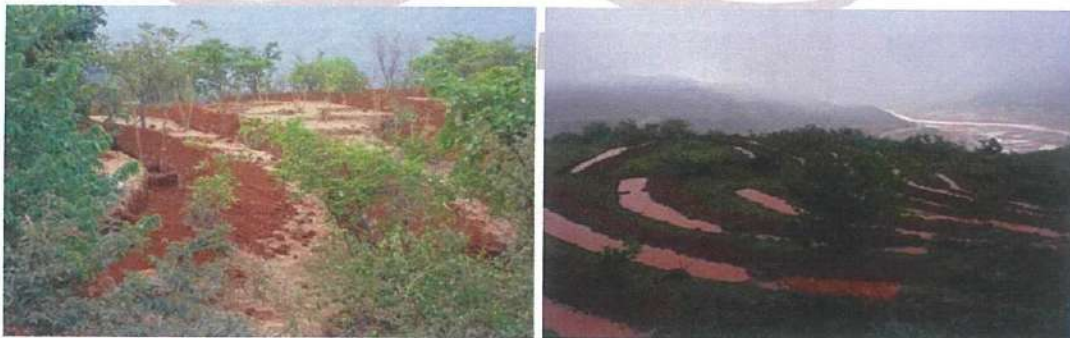
Fig 6.9: Continuous contour trench (CCT)
