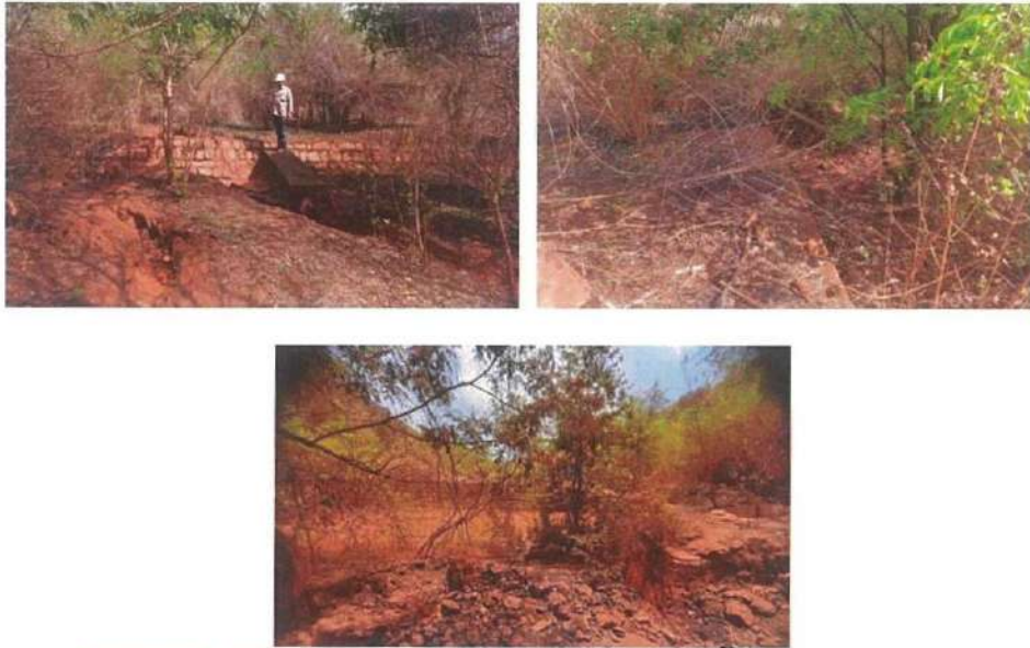
Fig 6.4: Existing Masonry structures at SMCP area.
