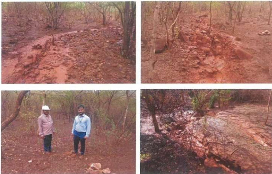
Fig 4.13: Proposed area for CCT & Gully plug in SMCP (To control the erosion).
