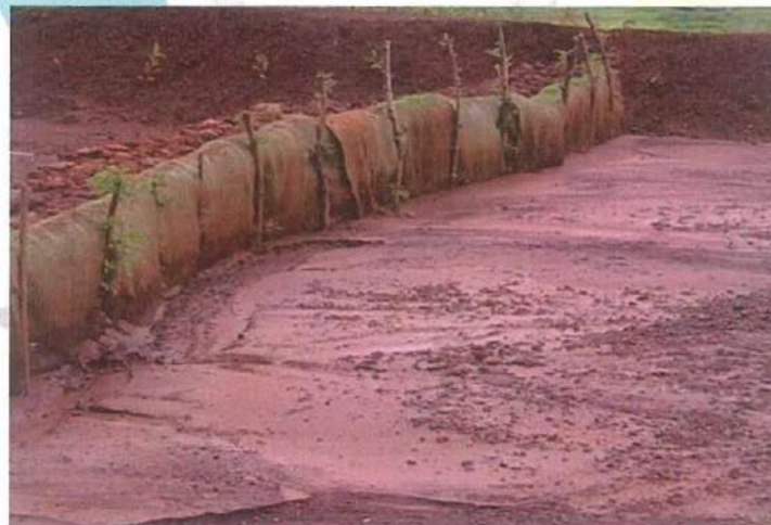
Fig 6.11: Geotextile Silt trap
