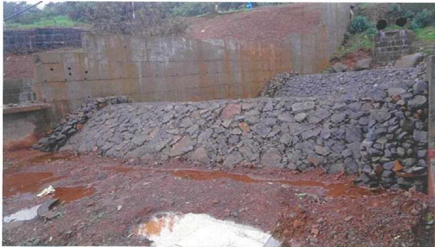
Fig 6.8: Large Gabion Structure
