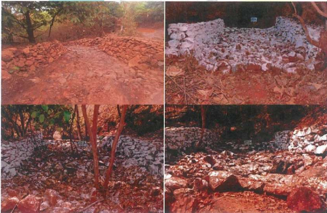
Fig 6.5: Existing Gully Trench structure at SMCP area.
