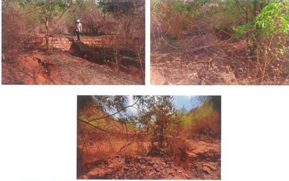
Fig 6.4: Existing Masonry structures at SMCP area.
