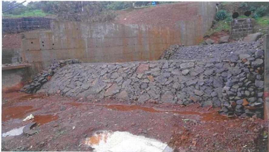
Fig 6.8: Large Gabion Structure
