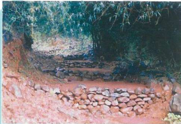
Fig 6.6: Gully Plug structure
