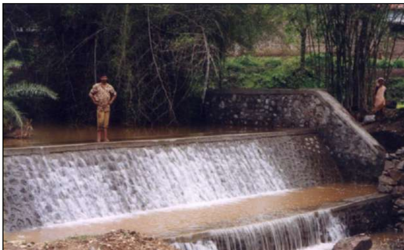
Figure 4: Masonry Check dam
