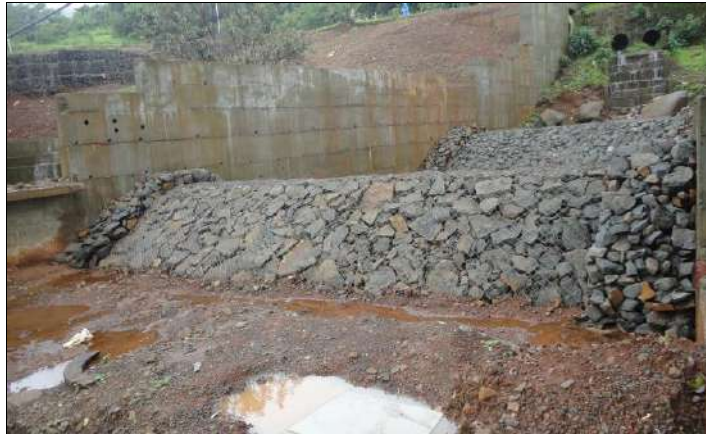
Figure 3: Large Gabion Structure with Chain Link
