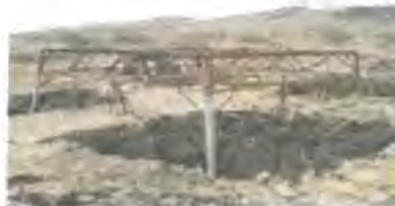
Stub setting & Template Assembly
