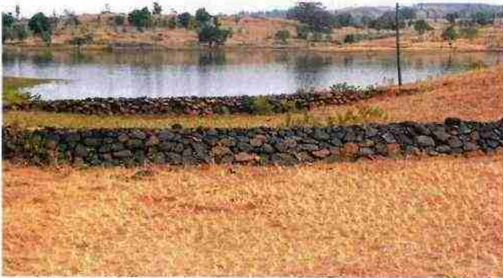
Loose Boulder Structures
