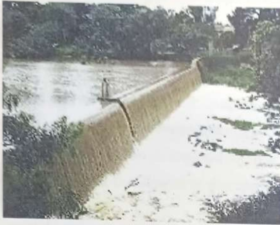
Photo showing the permanent weir
