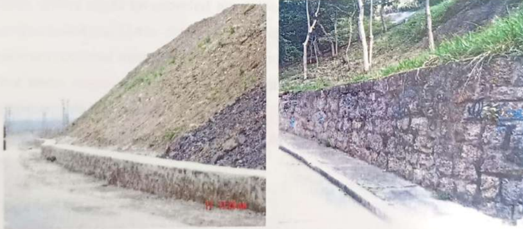
Photo showing the toe wall
