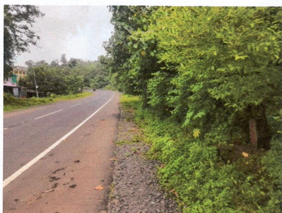
Ch. 31+840 (Left) pole 418
