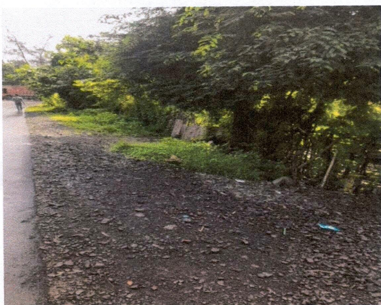
Ch. 22+350 (Right) pole 101
