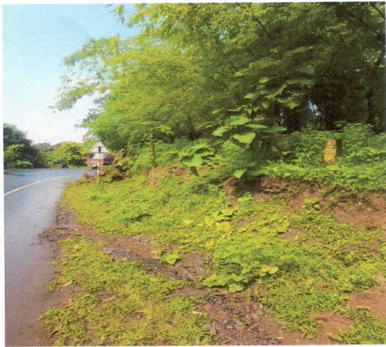
Ch. 22+350 (Left) pole 101
