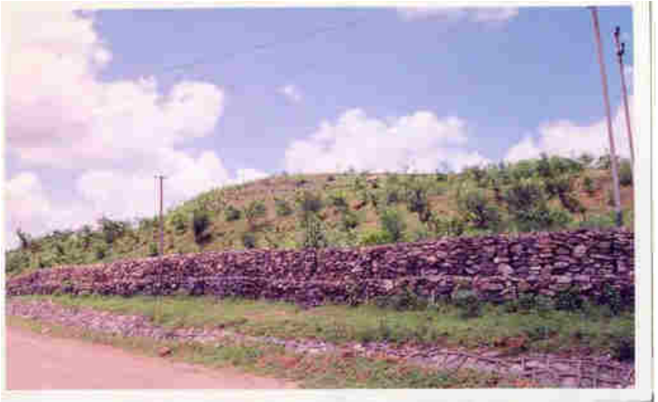
Fig. Gabion structure
