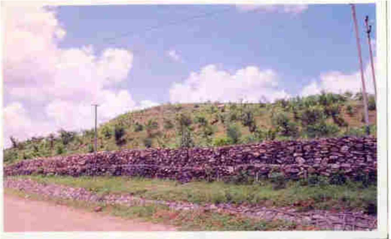
Fig. Gabion structure
