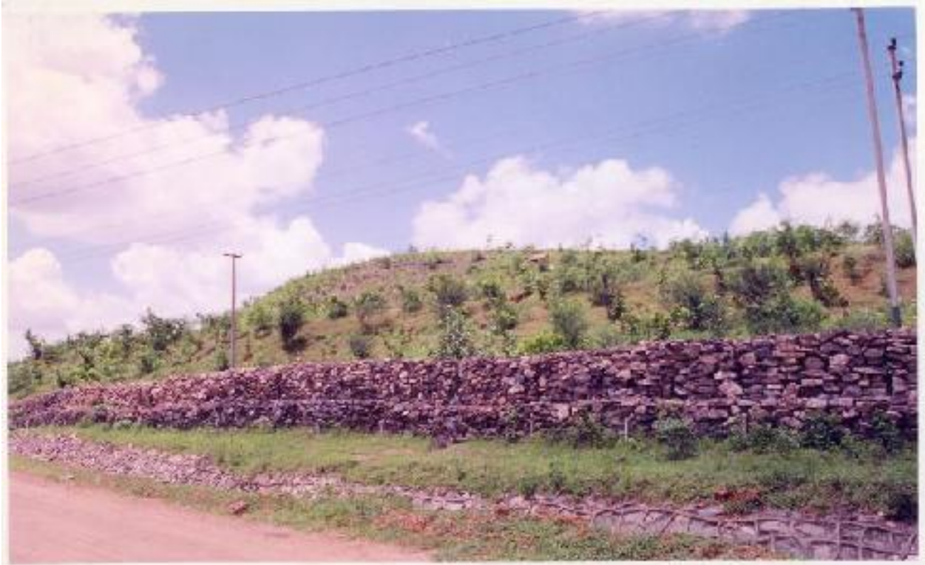
Fig. Gabion structure
