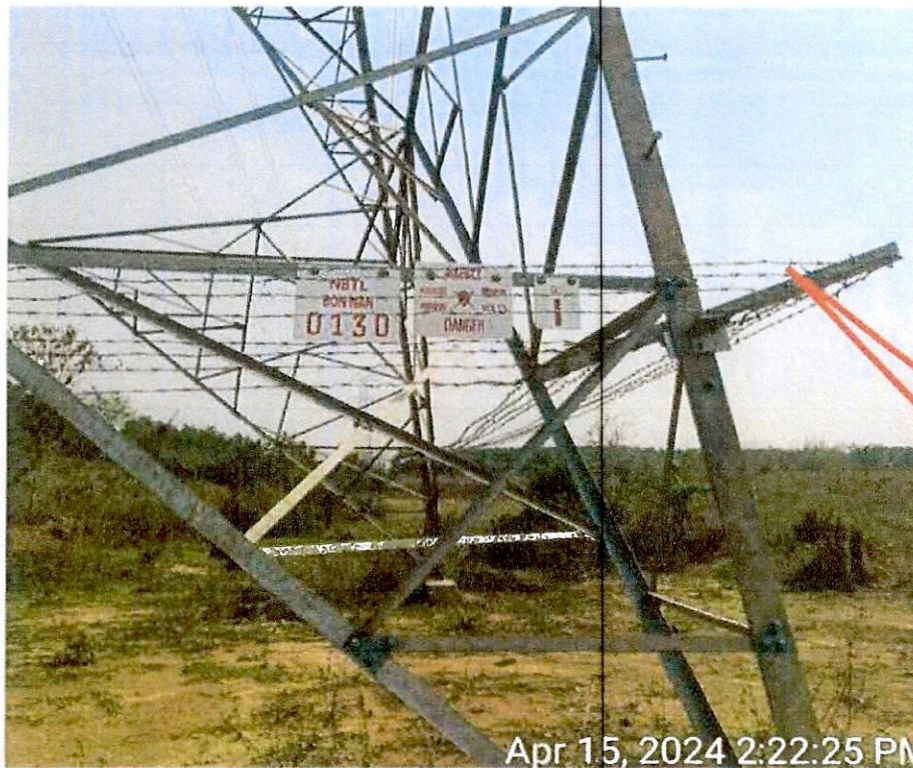
Anti-Climbing Device with Barbed wire Fencing
