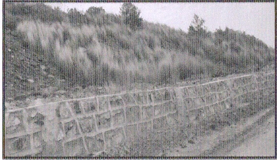
b. Along the Honhe OB dump, toe wall of 2 km length has been constructed.
