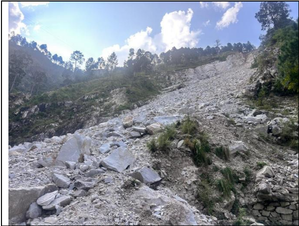
Site for crusher
