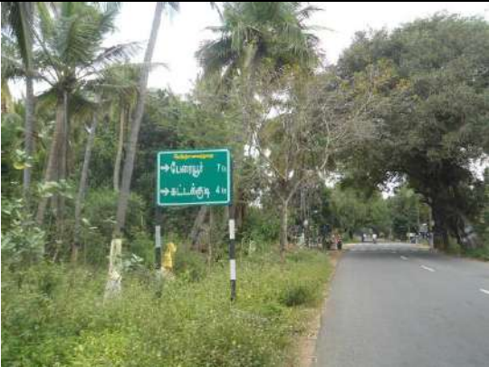
Pavement Condition at km 21+000
