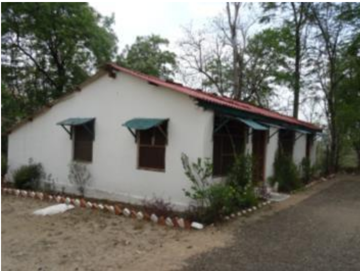
Photograph-08: Dhanora Forest Rest House
