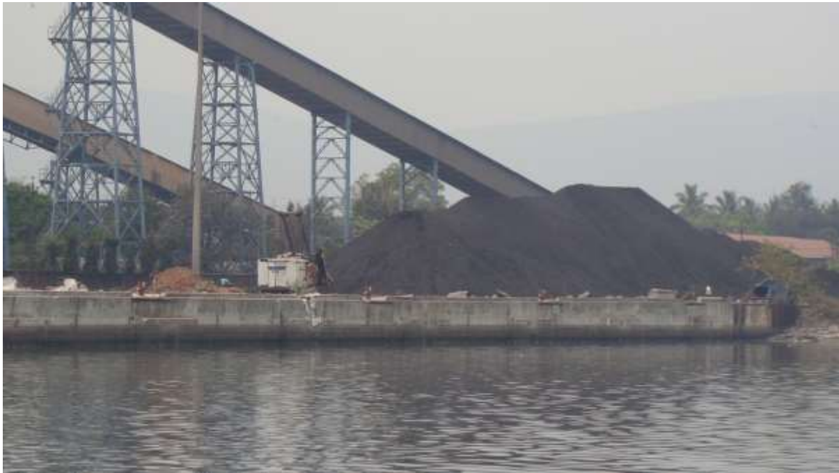
West Q-1 Iron Ore Berth
