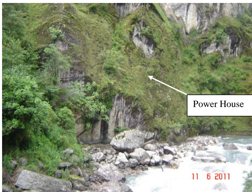
Photo 3-2 Area of the proposed underground Power house
