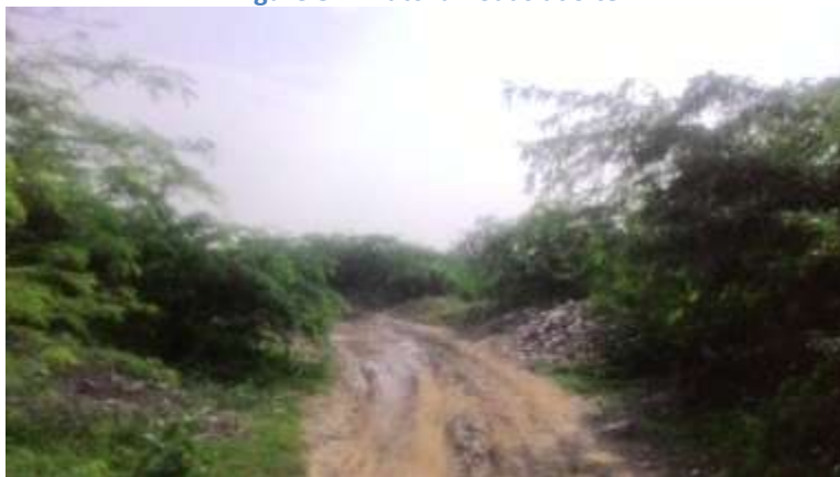
Figure 8-7: Kutcha Roads at Site
