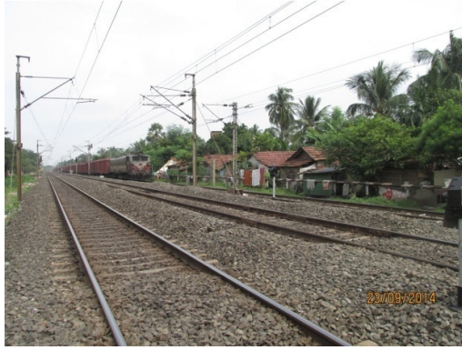
ENCROACHMENT AT DANKUNI
