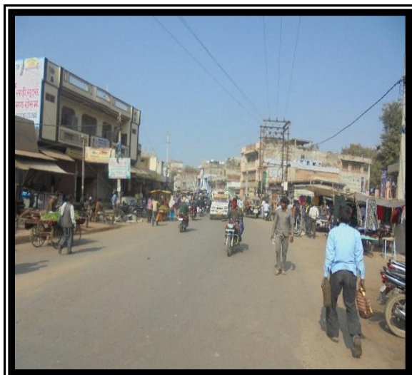
Photo-; Pavement Condition at Built-up Section
