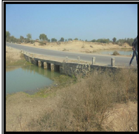
Slab Culvert at CH-15+000
