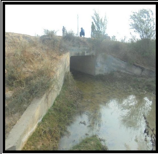
Slab Culvert at CH-2+760
