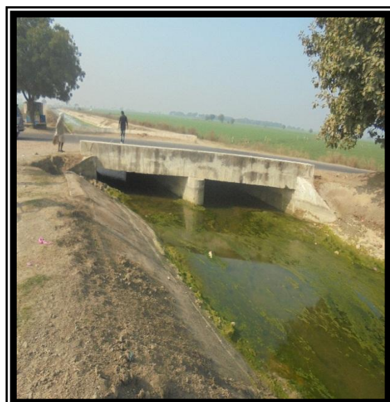
Minor Bridge at CH-10+010
